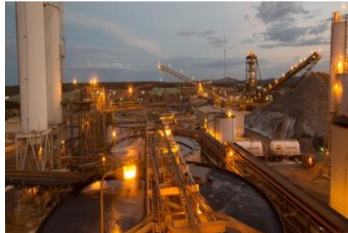
Golden Grove right size project underway.
